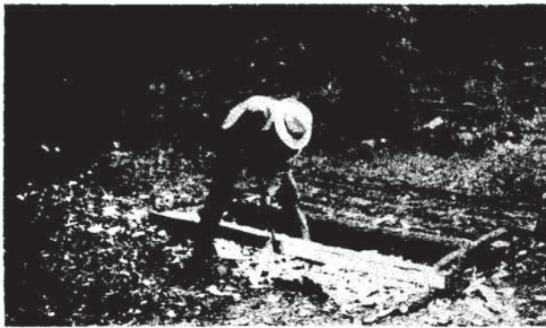
Fig. D.17. Hewing flat sides on a pole with a sharp ax.
