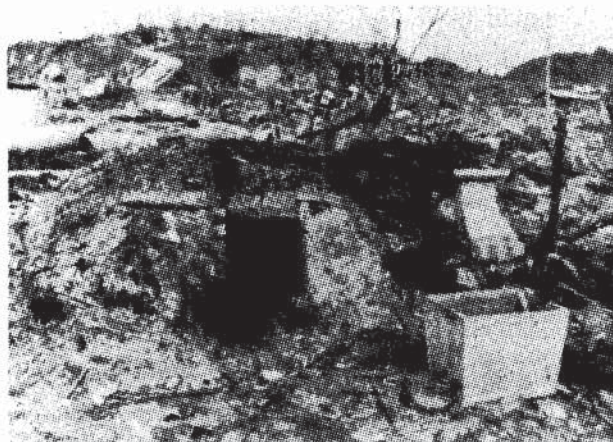
Fig. 1.5. Undamaged earth-covered family shelter in Nagasaki.
