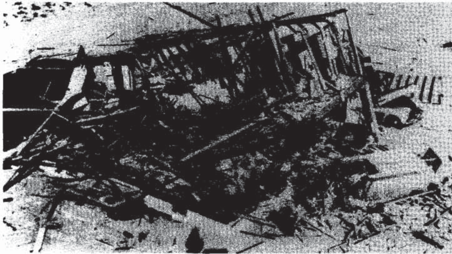
Fig. 7.4. Unburned wreckage of the same two-story, wood-frame house pictured in Fig. 7.1 after being wrecked by the 5-psi blast effects of a small nuclear test explosion.
