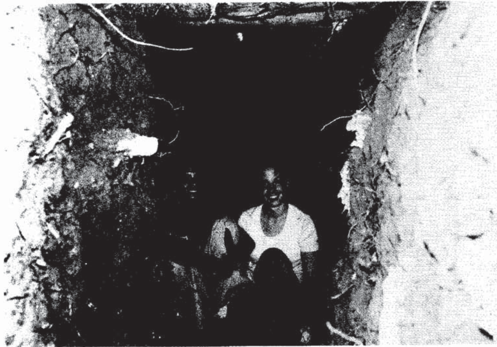
Fig. 5.2. Two non-athletic college girls who completed a 4-person Pole-Covered Trench Shelter in 35\frac{1}{2} hours, despite tree roots.
