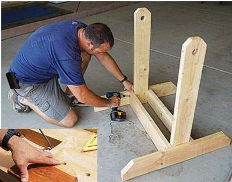
Above: Attaching the spacers to the two frame halves.
