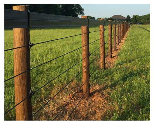
Electrifying your fence doesn't mean making the whole thing electrified, but rather adding an electric fence element to it. This is usually a single uninsulated wire, mounted
